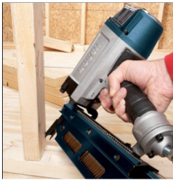
Toe nailing with a nail gun.
