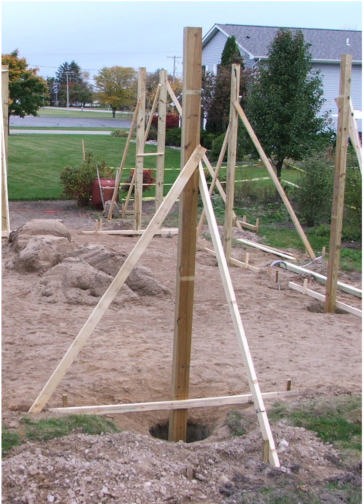
Photo shows columns suspended in holes by 2x4 horizontal.
