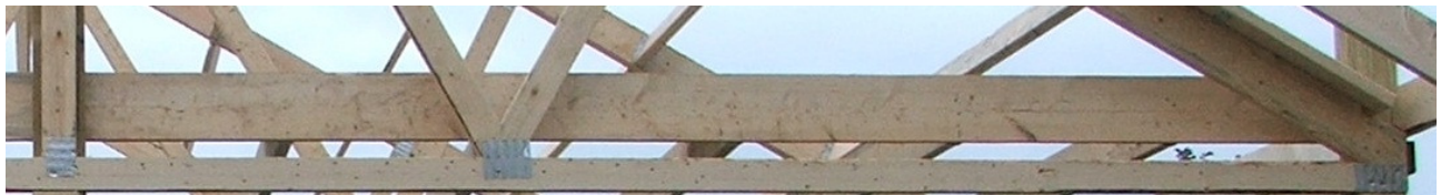
Ceiling end beam viewed from outside of building
